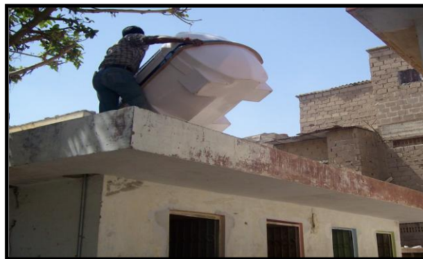
250 liter fiber over head tank being installed on the toilets building
