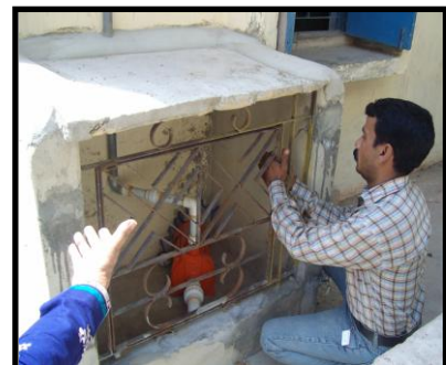
Plumber locks the motor after installing
