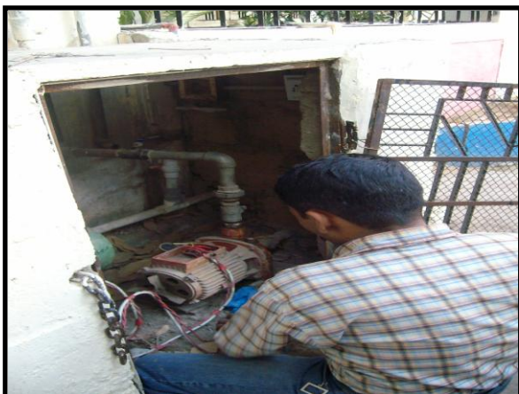
Electrician cum plumber repairs two broken down water pumps motors of Meridian Girls Secondary School
