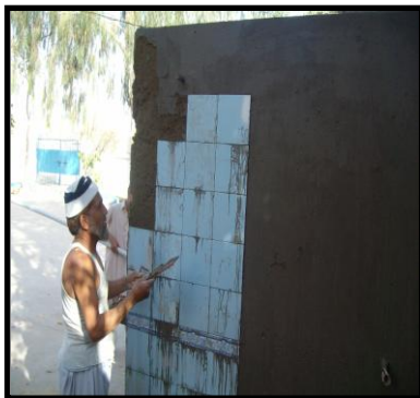
Mason fixing tiles on the new drinking water tank
