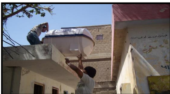
Overhead Tank being fixed on the toilets
