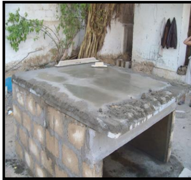
A new Drinking Water Tank being constructed by masons in the school compound
