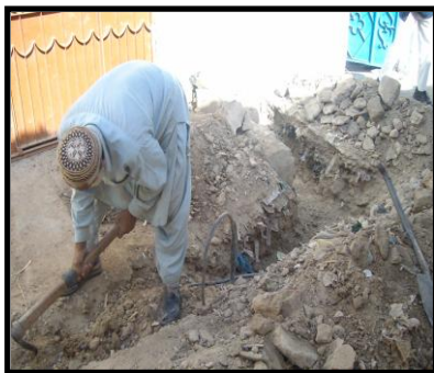
A labourer busy digging for sewerage pipe line for disposal of waste water from the toilets
