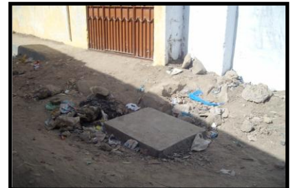
6 Chambers inside or and out side the schools reroute the main sewerage line
