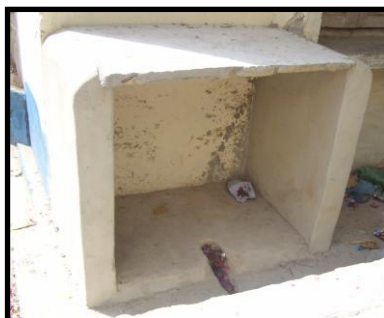
A cement cabin for electric water pump safety
