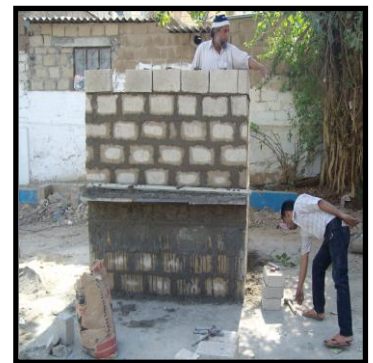
A new Drinking Water Tank being constructed by masons in the school compound
