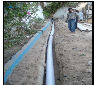
Sewerage line installation
