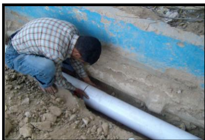
Plumber installing sewerage line
