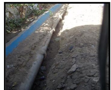
Sewerage line connected to main line
